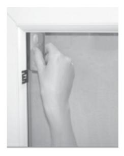
To line up the brackets, place a credit/store card vertically against the glass at the top of the window. Where the bottom of the card sits, this is the installation point for the first bracket. Install all of the brackets provided, installing any intermediate brackets accordingly.
